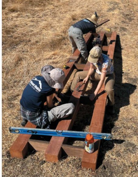
Staff build a bridge for an ephemeral stream at Mangini out of reclaimed old-growth redwood.
